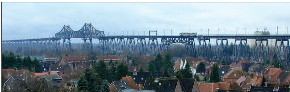
Fig. 1: Rendsburg High Bridge with the “canal bridge” (the main bridge, left) and the “loop bridge” (right)
