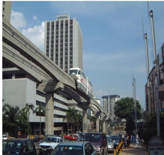
Fig.1: KL Monorail Car on Guideway Beam
