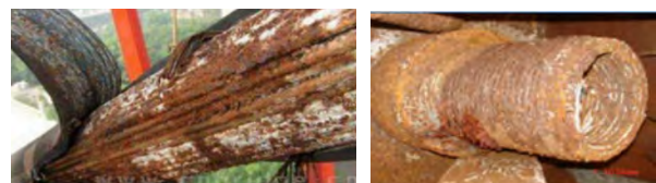
Figure 1. Corrosion of cable wire and anchorage
